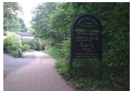
Thurgoland Tunnel ahead with new Trail surface
